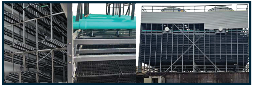
SPLASH TYPE COUNTER FLOW COOLING TOWER
